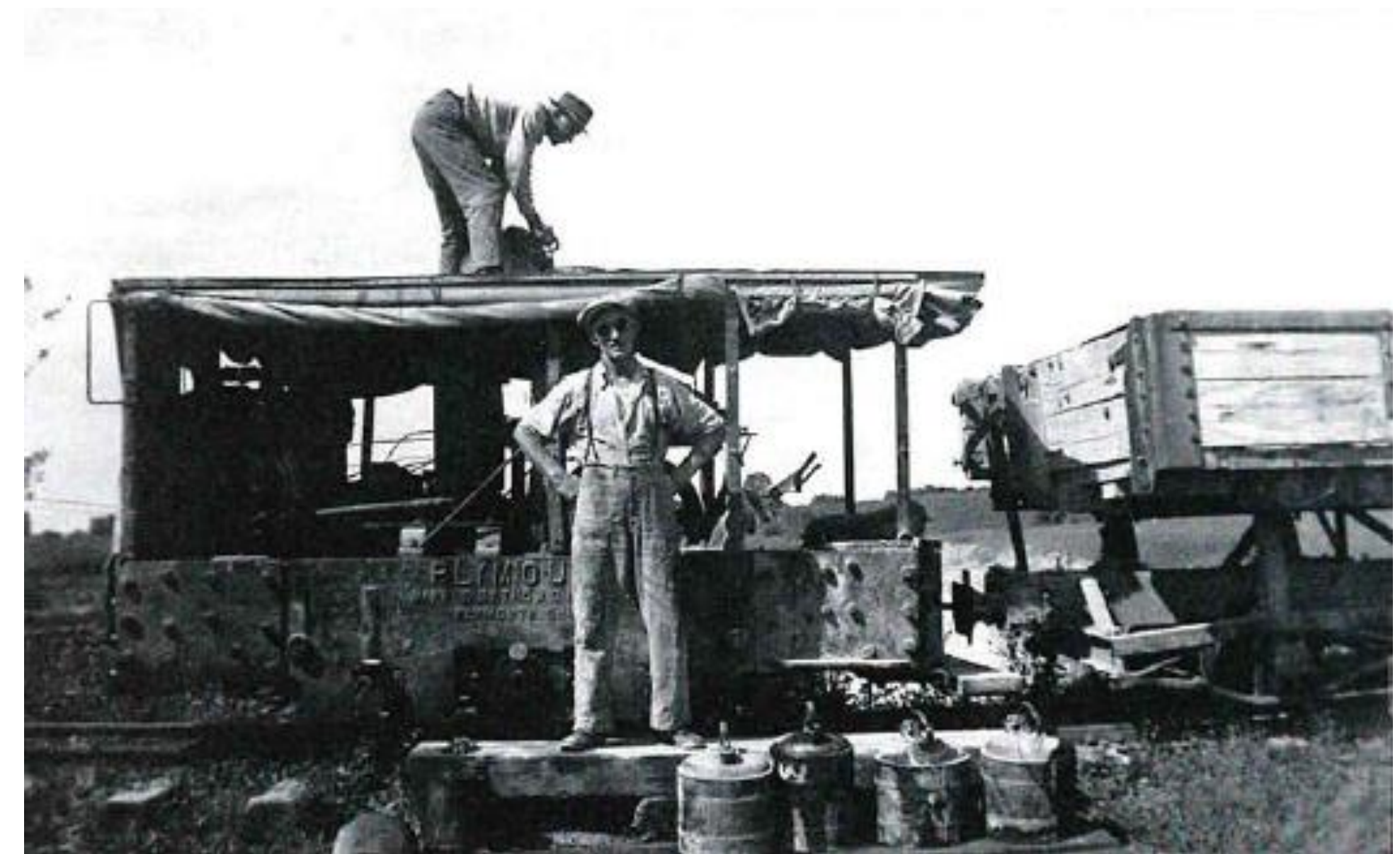
Refueling the Plymouth locomotive used on site for material transfer
