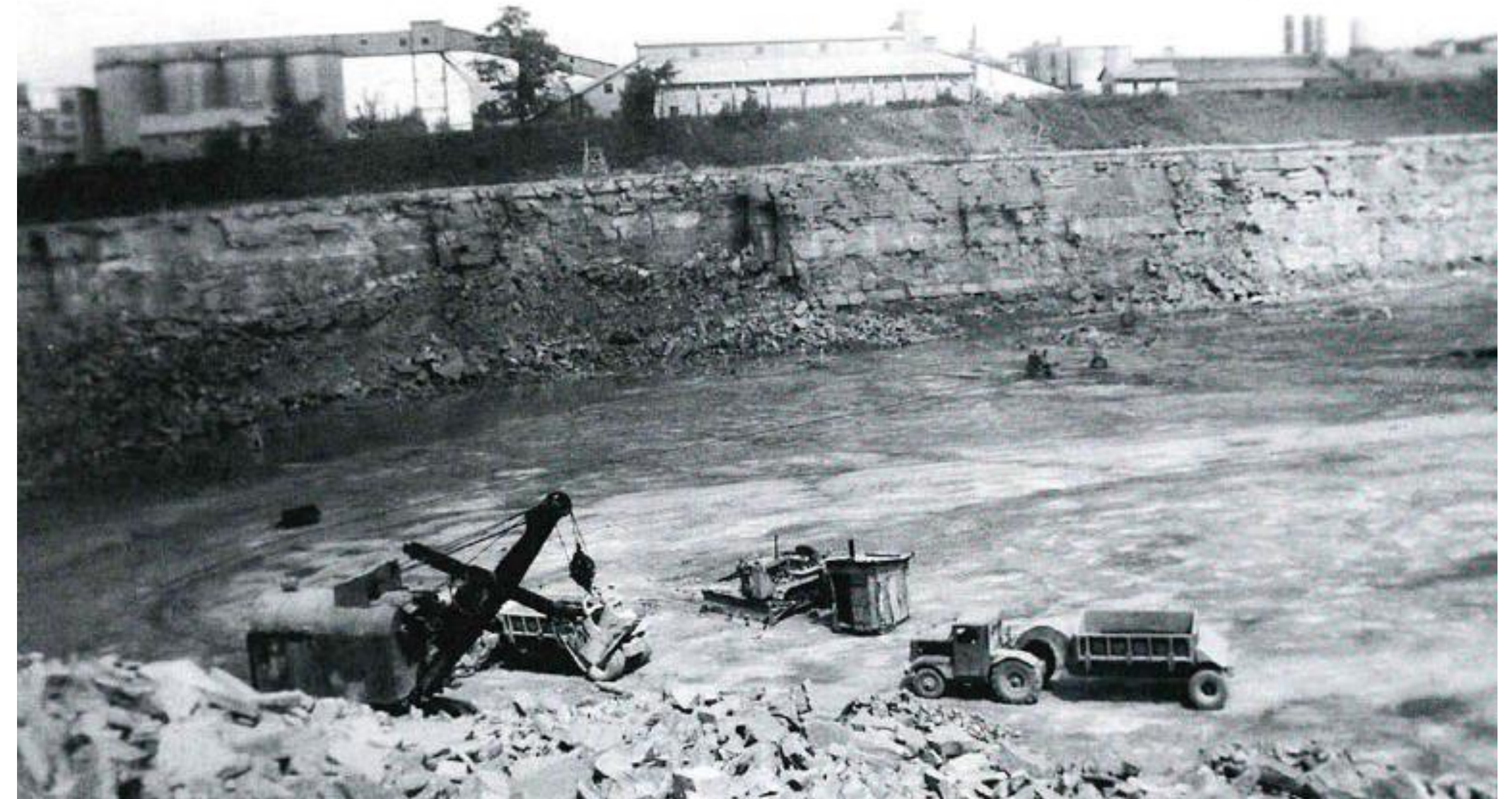
Electric shovel with truck and side-dump trailer in the stone quarry, 1940s.
