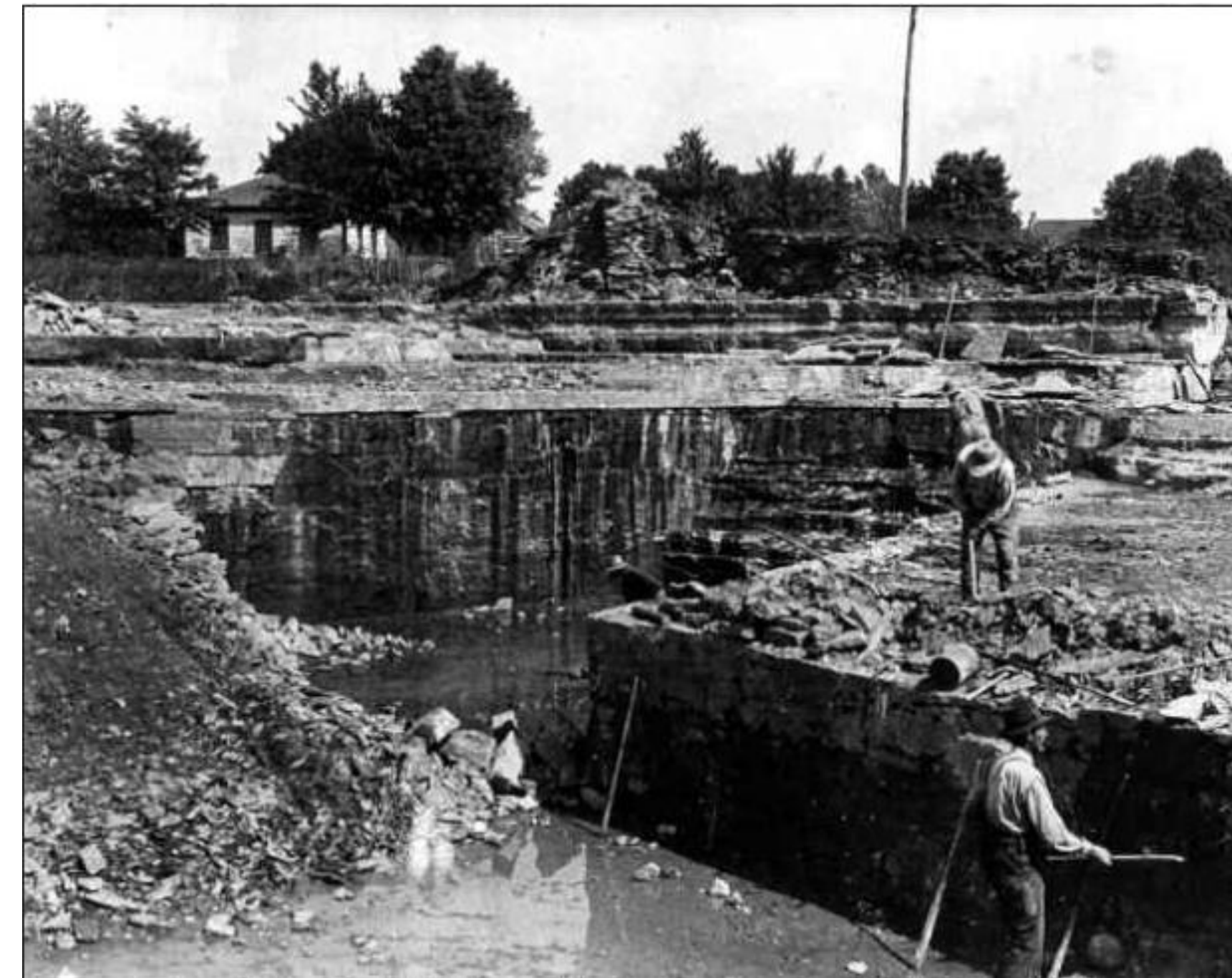
"Quarrymen work in the Thames Quarry beside Water St". 1904. They are using centuries old methods to extract blocks of limestone from the sedimentary layers in the quarry.
