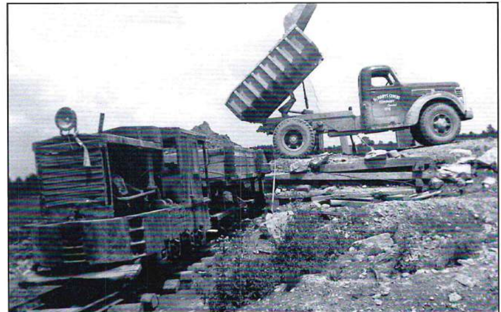
A truck dumps a load (probably of clay) into a cart drawn by one of the Plymouth Locomotives used for decades in the cement plant. These engines were comparatively small and ran on narrow-gauge tracks. Gord Foster collection, courtesy Ann Switzer
