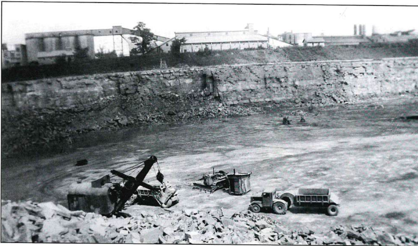
Electric shovel with truck and side-dump trailer in the stone quarry, 1940s. Gord Foster collection, courtesy Ann Switzer
