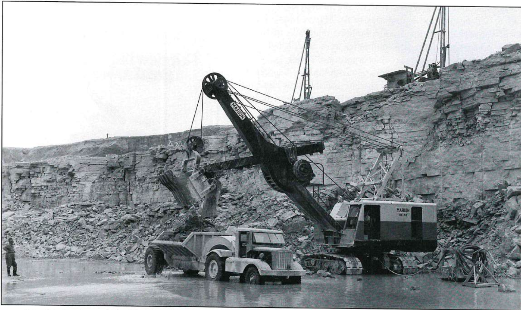
According to notes made by John King, this undated photograph shows No. 2 Quarry with a Marion electric shovel and side dump. Two Joy drills are in the background. St. Marys Cement Company collection.
