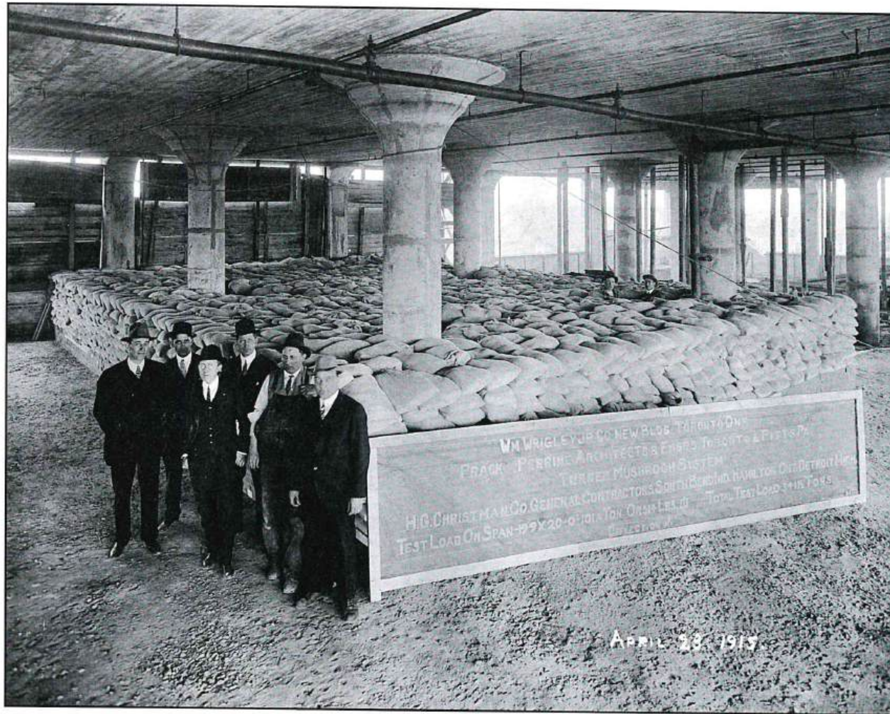
Testing the floor load capacity in the Wrigley building, 1915. Today this building has been converted into loft-style condos. Advertising emphasizes the original warehouse windows, the 14-foot ceilings and the gigantic concrete mushroom pillars visible in this photograph. Laidlaw Collection, St. Marys Museum
