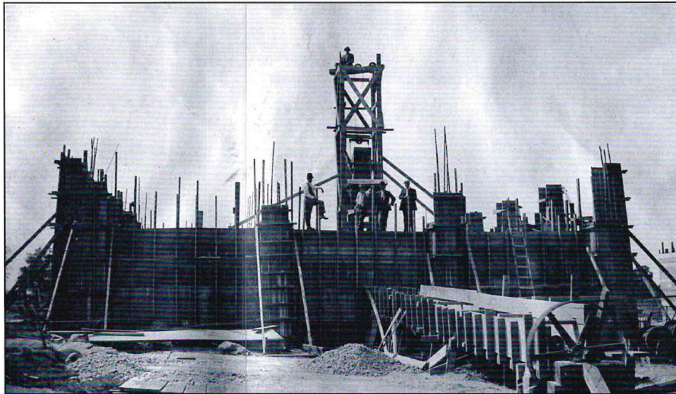
The main buildings were made of cement. This photograph shows the grinding mill taking form. Laidlaw Collection, St. Marys Museum
