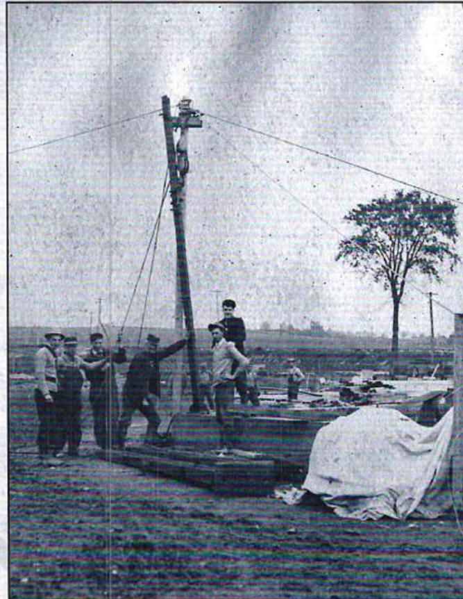
Erecting hydro poles into the cement plant Laidlaw Collection, St. Marys Museum
