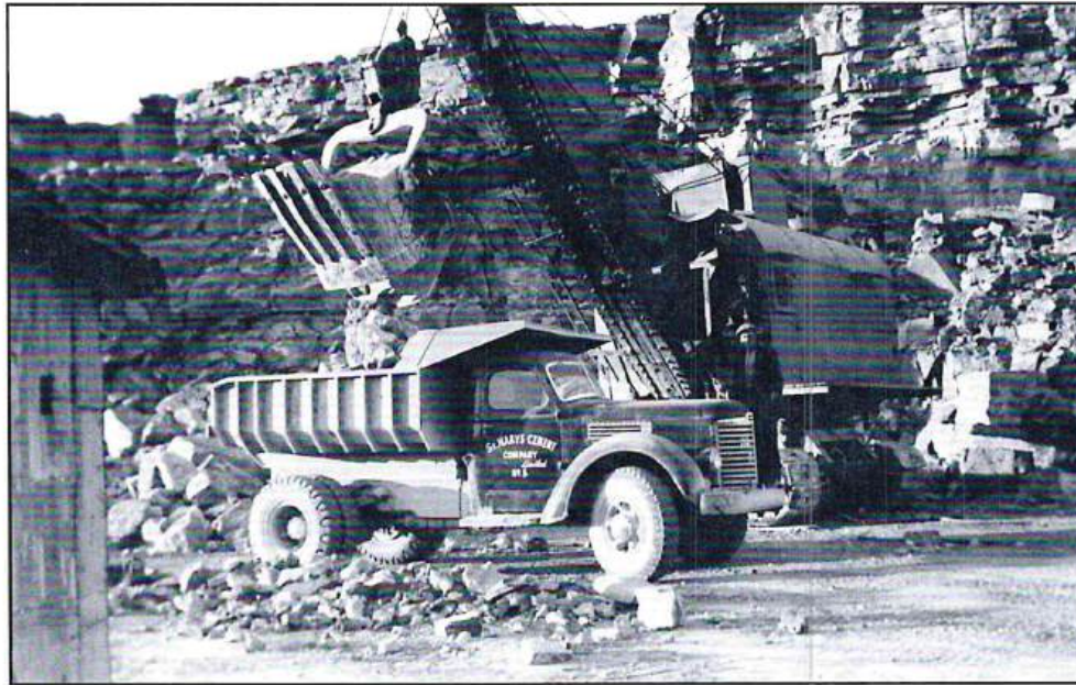
An electric shovel is used to load stone into a truck in the quarry. Gord Foster collection, courtesy Ann Switzer
