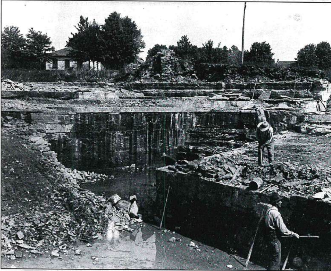
Quarrymen work in the Thames Quarry beside Water Street in St. Marys in 1904. They are using centuries-old methods to extract blocks of limestone from the sedimentary layers in the quarry. St. Marys Museum collection
