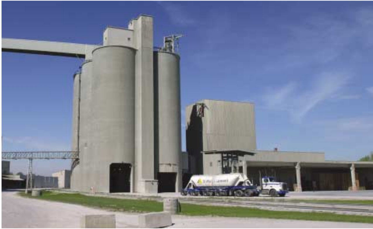
The St. Marys plant has 90,000 tonnes of cement storage while production capacity is more than seven times that amount.
