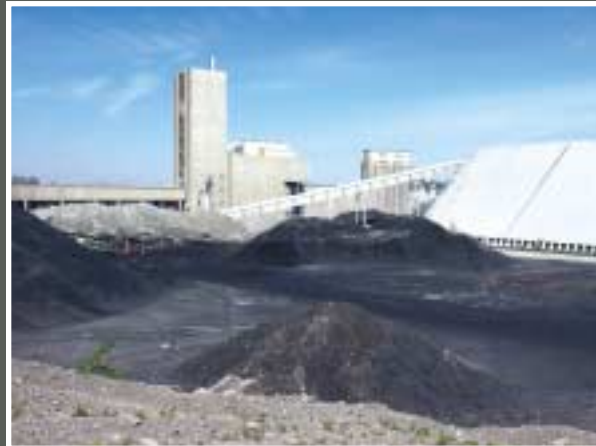
Coal and coke are stored in the yard until required as fuel.
