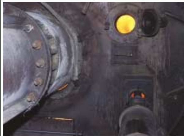
Using a mixture of coal and coke mixed with air for fuel, cement kiln temperatures reach 1870^{\circ}\text{C} causing a chemical change in the raw material.
