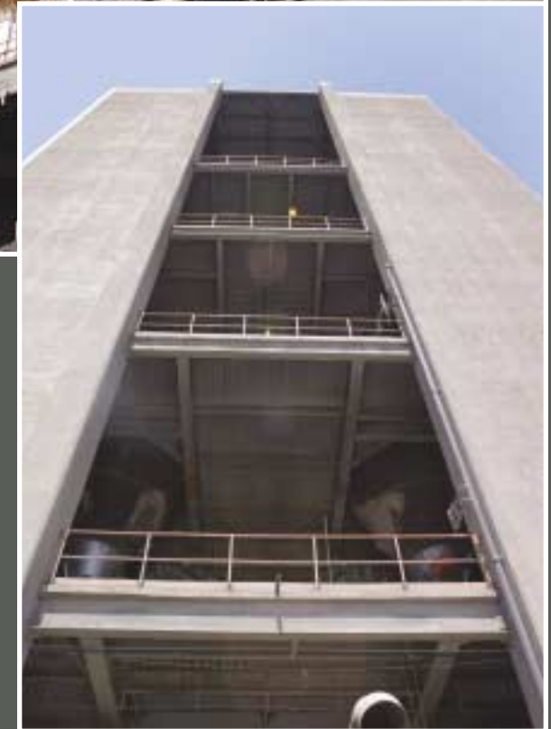
The four stage preheater tower uses waste heat from the kiln to raise the temperature of the raw meal and reduces the energy required to produce the clinker.
