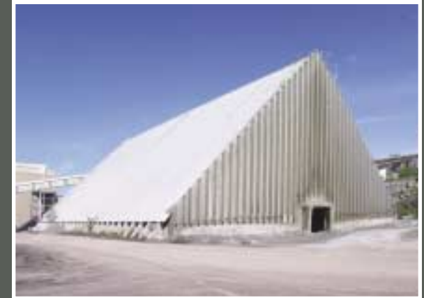
The A-frame storage building is used for the storage of clinker until it can be ground.
