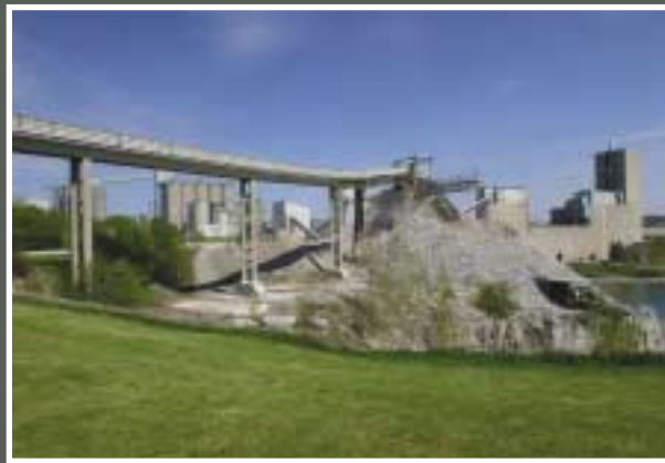
An extensive conveyor system moves raw material from the primary crusher in the quarry to the stockpile near the plant.
