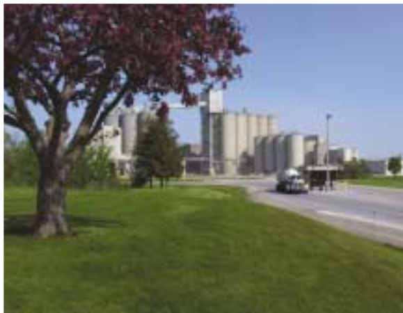
Gate No. 1 at the St. Marys Plant
